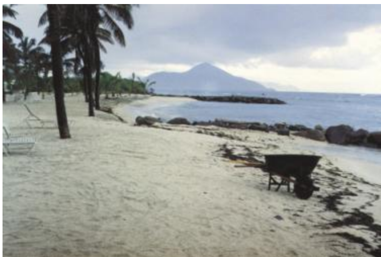
Groyne at Nisbett Plantation, Nevis. The sand has built up on the updrift side of the groyne in the foreground, while the waves reach further inland on the downdrift side as a result of erosion.
